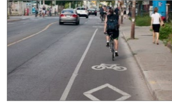
Painted bicycle lane
