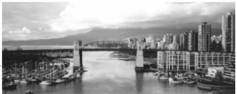
Burrard Bridge: too dangerous for safe non-motorized transportation?
